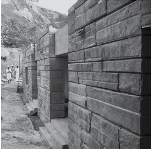
Reuse of excavated granite as a cladding material for Gota Dam
